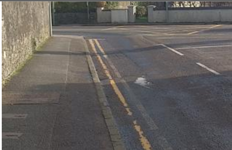
Figure 8.2 Photo Direction D
