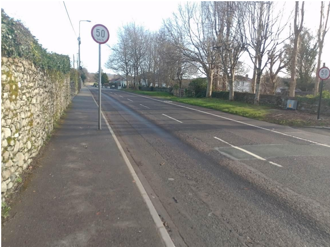
Photo A1 – Speed Limit Control along Ross Road
