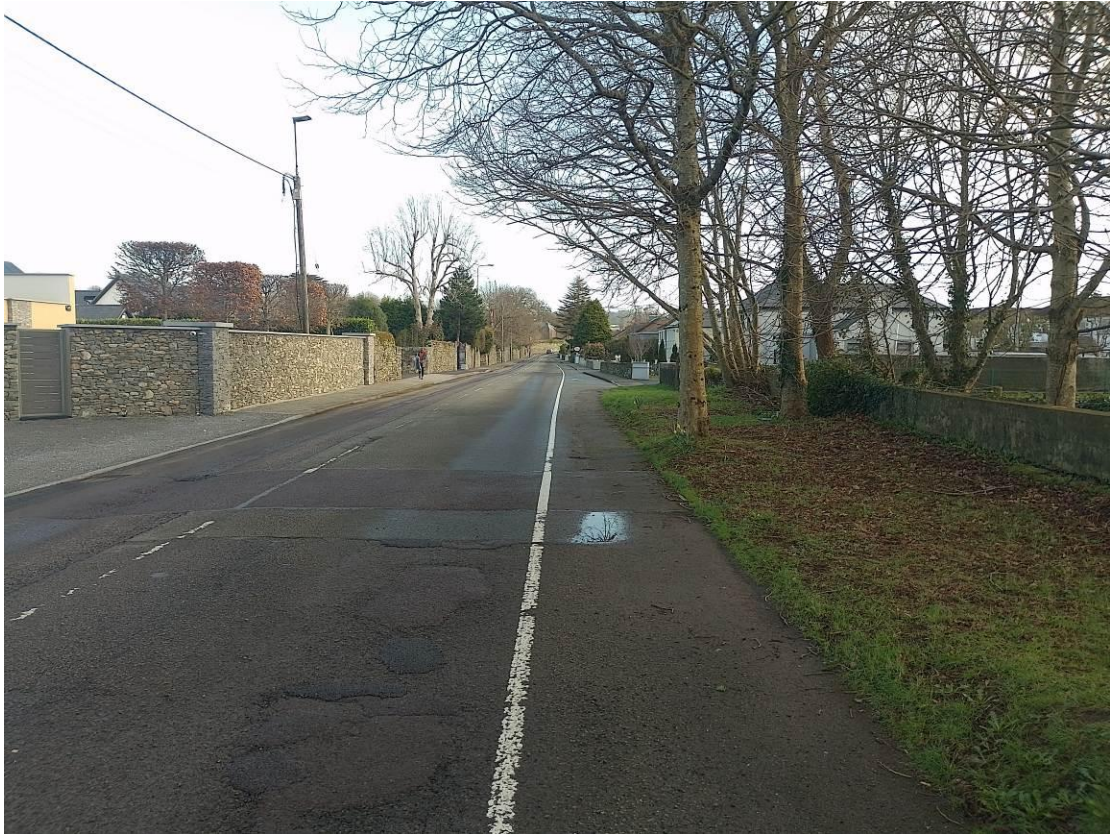
Photo A3 – Existing Sightlines to North of Proposed Vehicular Entrance
