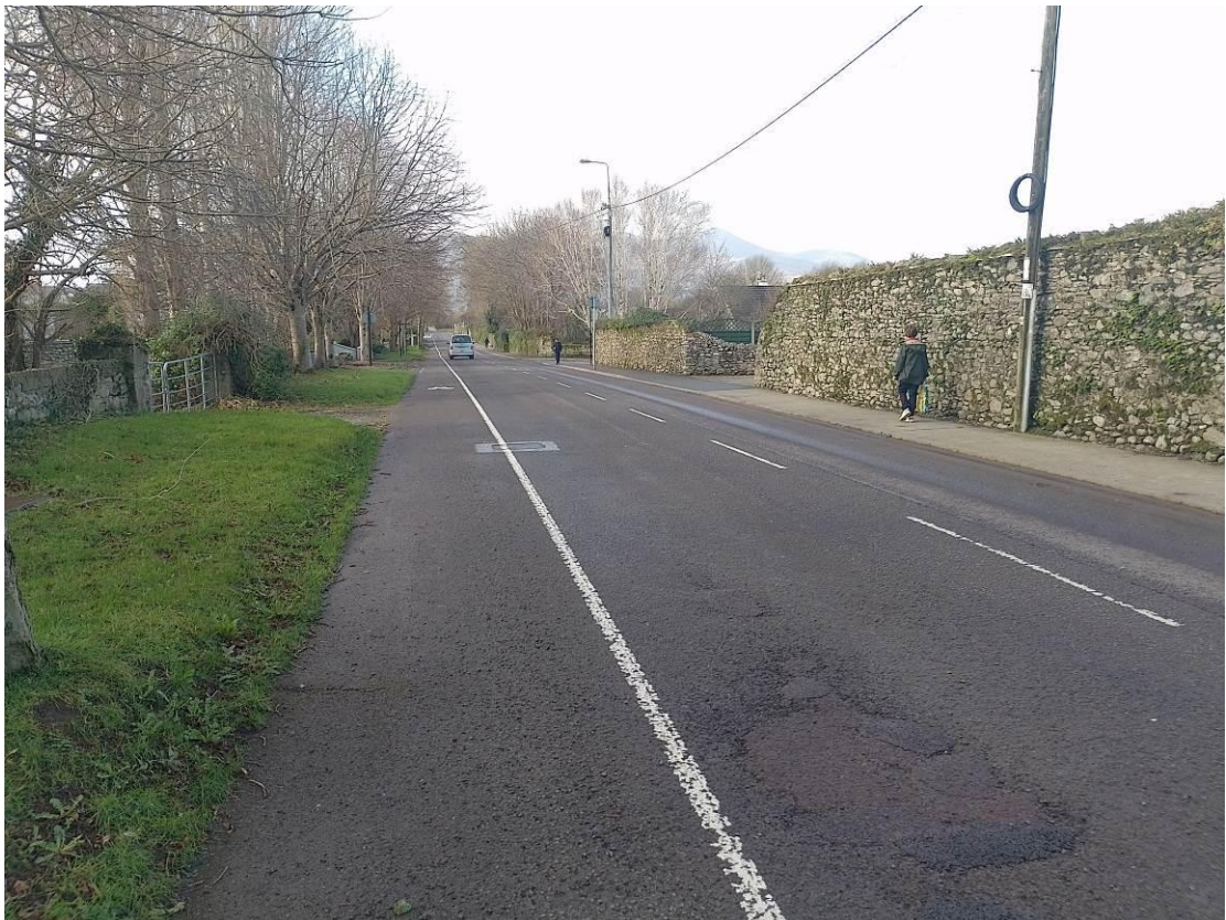
Photo A4 – Existing Sightlines to the South at Proposed Vehicular Entrance
