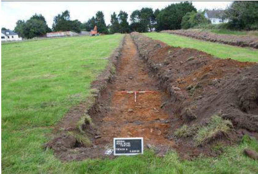
Plate 5: Trench 9, facing north
